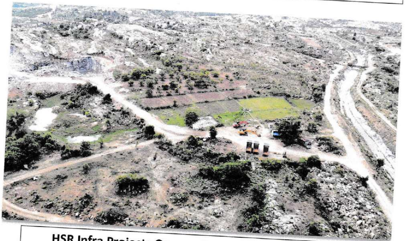
HSR Infra Projects Metal Crusher, Gudlanayanapalli Village, Kuppam, A.P
