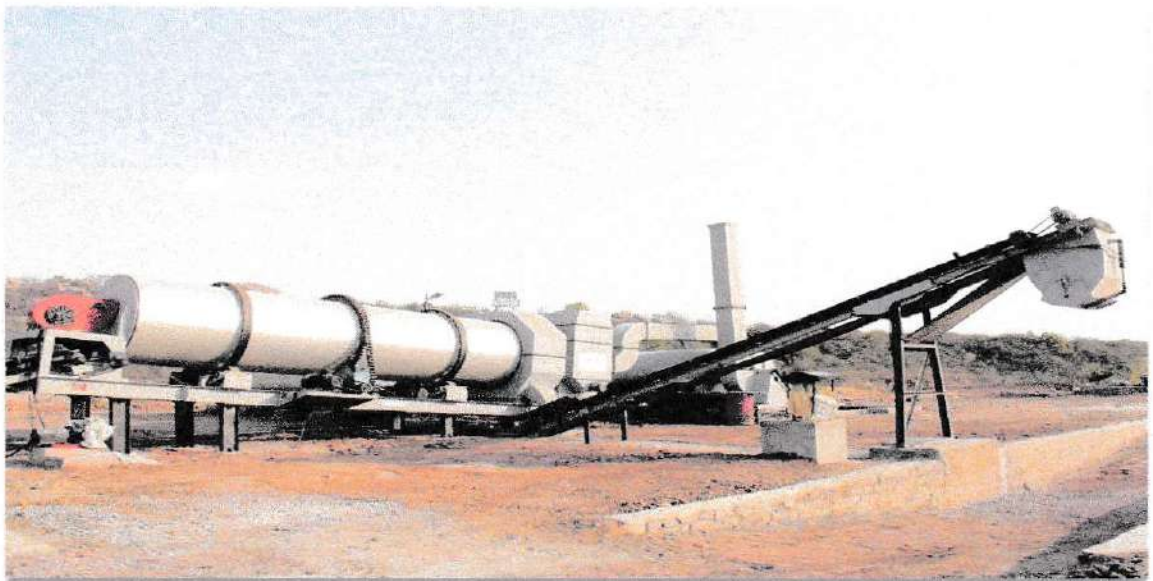
HSR Infra Projects Drum Mix Plant, Karampudi, Palanadu District, A.P
